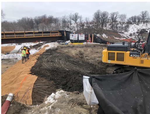
SF 35, photo facing west, excavator building up river bank on the other side.
