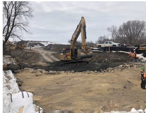
SF 35, photo facing south, excavator building up the river bank.
