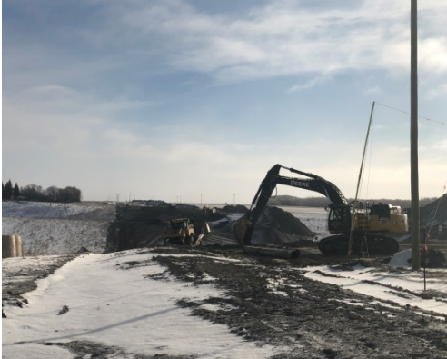
SF 40, photo facing east, two dozers and one excavator moving dirt.
