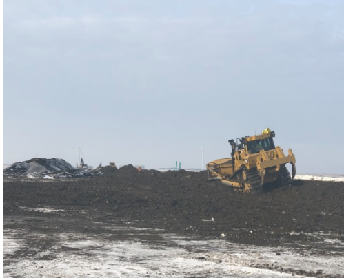
SF 50, photo facing west, two dozers and one excavator moving dirt on the ROW, smoothing/flattening it out.
